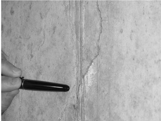
Cracks which are horizontal are most likely caused by an applied load. Vertical cracks which are significantly wider at the top or bottom could indicate heaving or settlement. With these cracks it is very likely that the crack itself is not the problem, but rather the result of an external problem such as poor drainage, overloading, etc.
