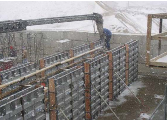
Fig. 2: Placement conditions for the full scale walls in Phase 2 included temperatures of 26°F and falling along with active frozen precipitation.
