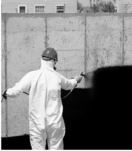
Fig. 4: Spray-emulsion waterproof coating applied to a concrete foundation wall.
