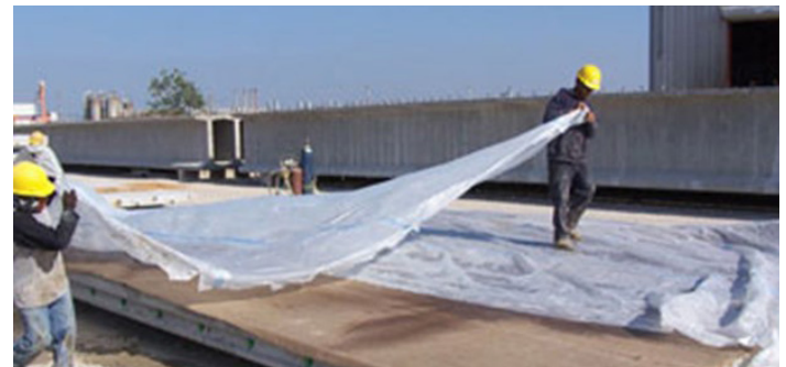
Fig. 10: Burlap and plastic curing.
