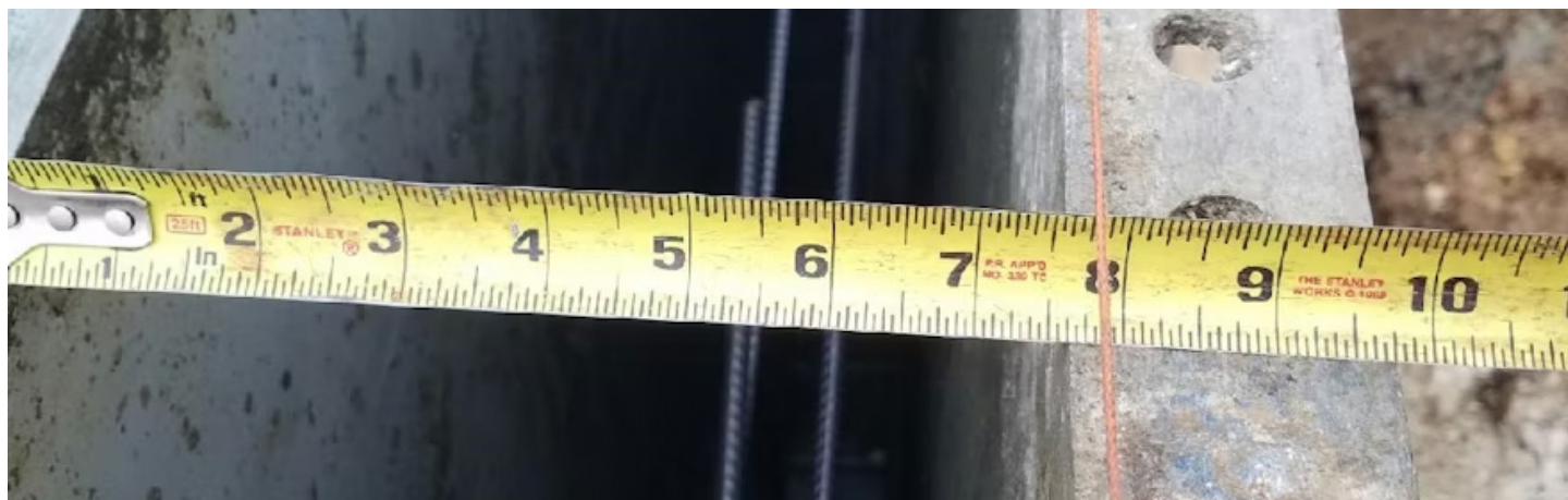
Fig. 1: Concrete wall forms set for residential foundation showing a nominal 8-in. wall thickness with an actual thickness set at 7 5/8-in. Concrete Foundations Assoc.
